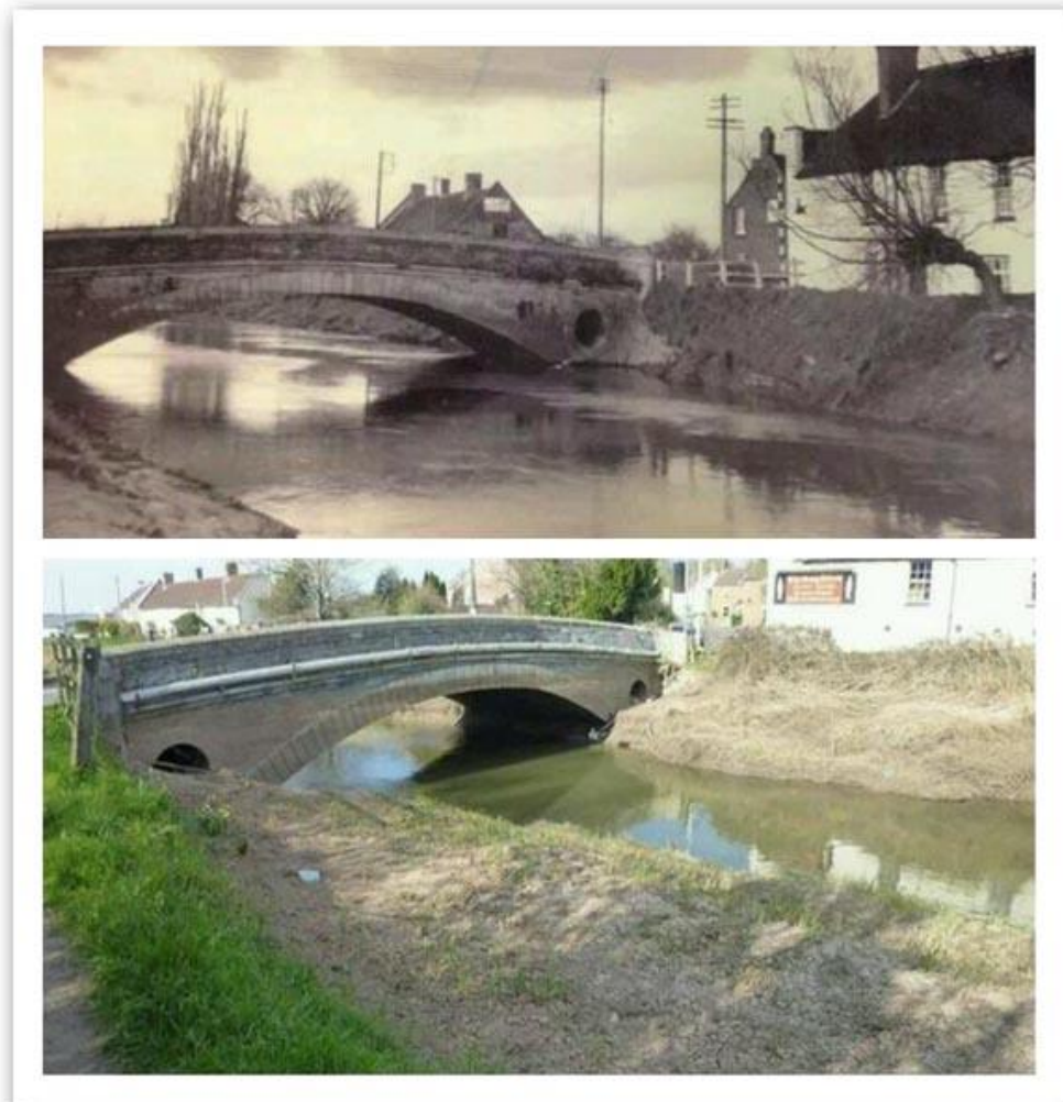
Figure 5: Even without the strategic effects of EU legislation, the Habitats Directive and the Waste Framework Directive were hindering dredging, requiring expensive pre-action assessments and increasing the cost of sediment disposal. The effect are evident at the bridge over the Parrett at Burrowbridge, the top picture taken in the 1960s and the other within the last years.
