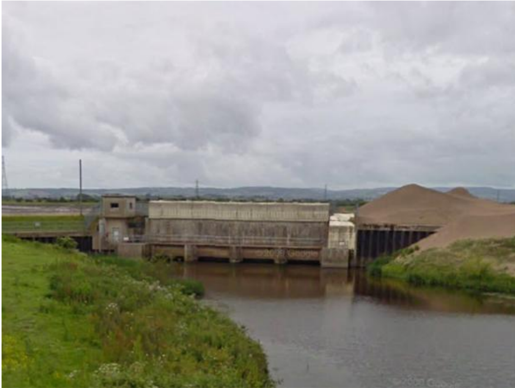
Figure 7: Dunball Clyce, taken from the Huntspill River Bridge on the Bristol Road, looking west, towards the Parrett Estuary.
