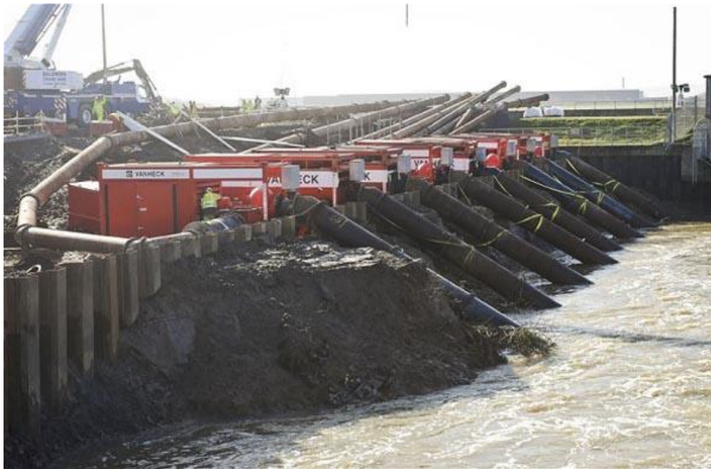
Figure 11: the Dutch pumps in action at Dunball sluice. Collectively, by early March, the pumps were moving 7 million tons of water a day.
